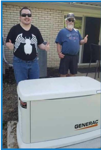
It's a thumbs up from Aaron Knight (l) and Bruce Hart for the whole-home generator at their Kenbrook home (RHA.)
